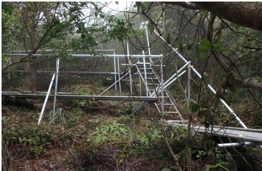
Plate 1. Vegetation clearance was kept at minimum for building temporary access to the transplantation receptor site.
